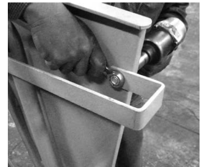
Figure 2-6 Headgate Guide Inside
