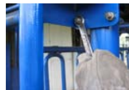
Fig. 3 Tightening Top Nuts
